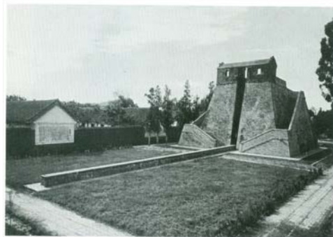
Fig. 116. The Chou Kung Tower at Yang-chhêng; looking along the shadow scale with its water-level channels (photo. Tung Tso-Pin et al. ).
