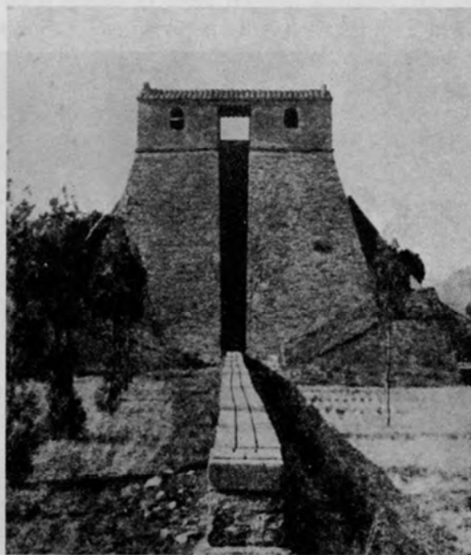
Fig. 116. The Chou Kung Tower at Yang-chhêng; looking along the shadow scale with its water-level channels (photo. Tung Tso-Pin et al. ).
